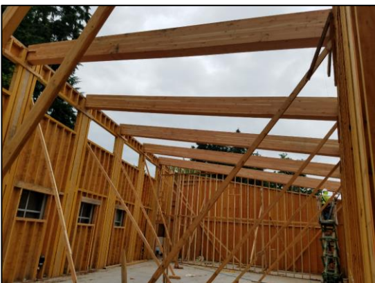
Police Station Addition
